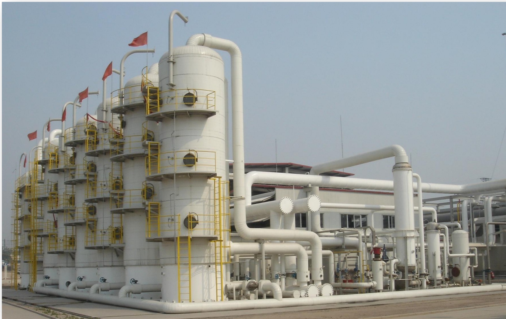
35,000 Nm 3 /h PSA-H 2 Unit from COG in Shanxi
