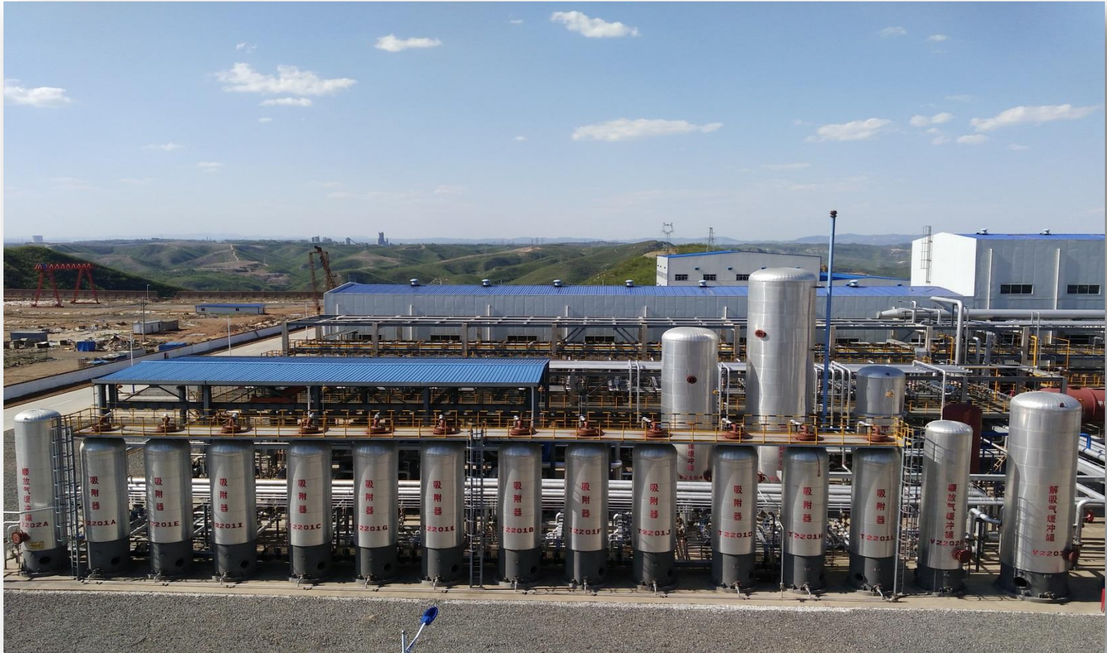
170,000 Nm 3 /h PSA-H 2 Unit at Shenhua Ningmei Indirect Coal to Oil Complex
