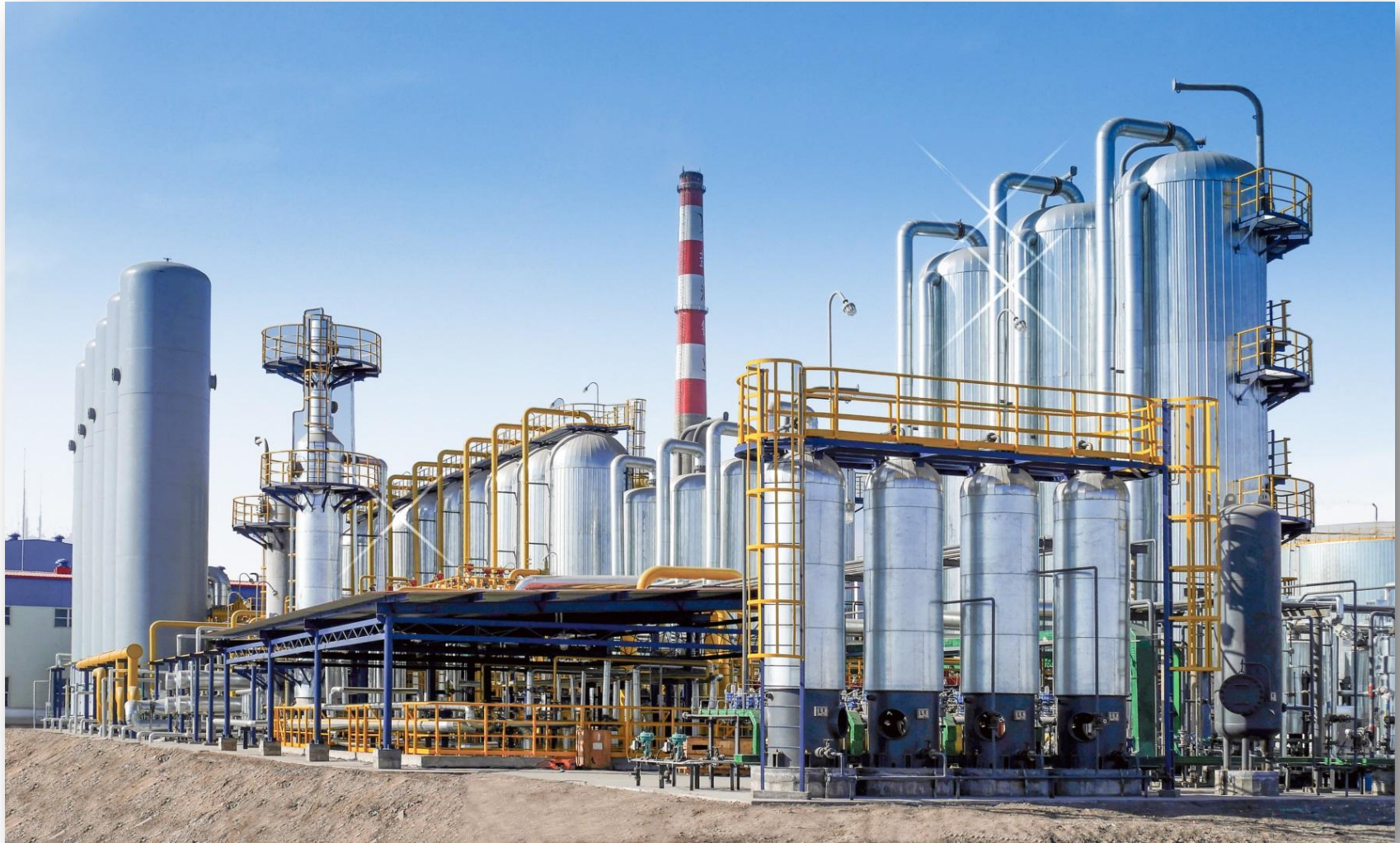
140,000 Nm 3 /h PSA-H 2 Unit from COG at Qinghai Salt Lake Company
